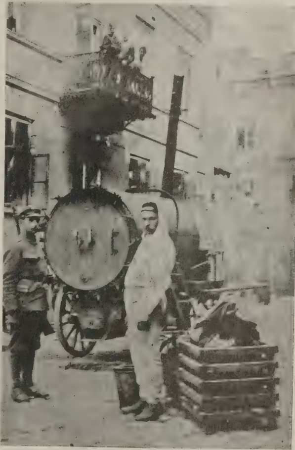
Courtyard of a crowded Warsaw tenement, showing a disinfesting plant in operation
